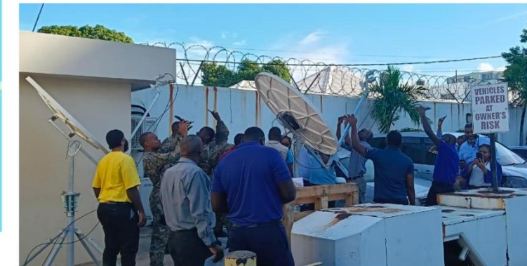
Fixed antenna installation training
